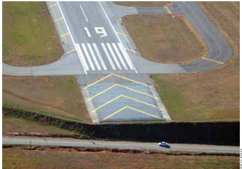
The “crushable concrete” beyond Runway 1 in Greenville, S.C., could prevent a nasty plunge during an overrun.
